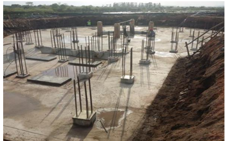
WTG Piling Work
