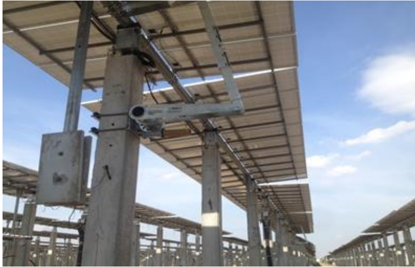
Motor Tracker Installation
