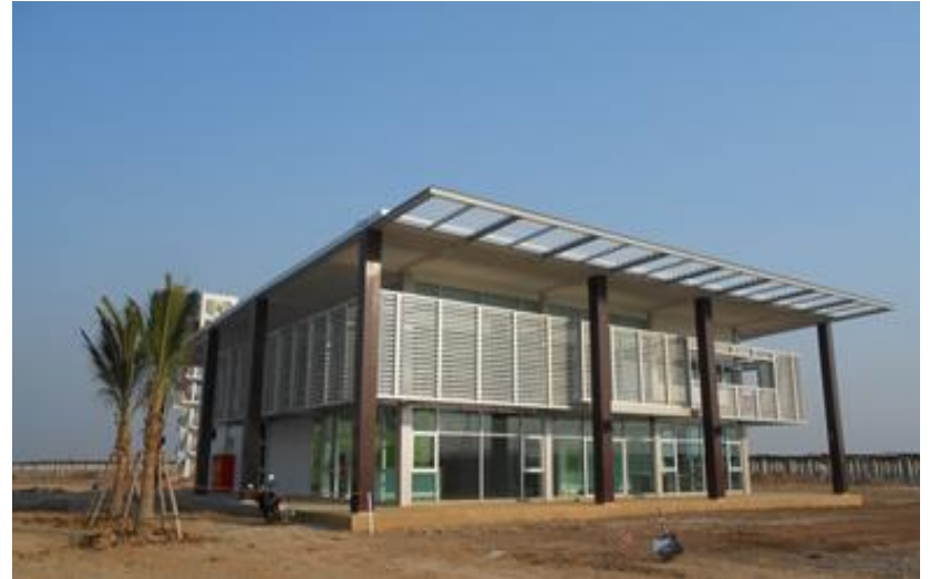
Control Center Building
